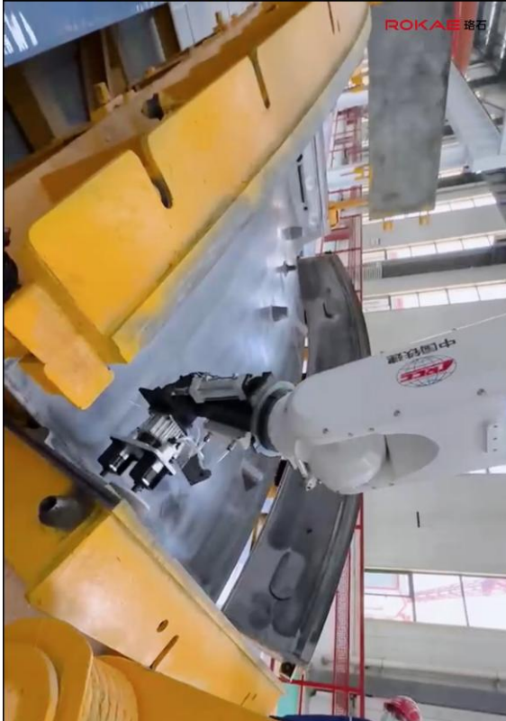
Tunnel cement segment mold grinding
